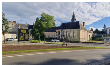
Photograph Almatoya Architecture 12/08/2025 – Loire-et-Cher – Blois Post Office Work on the post office was pushed back to the second half of the 1950s. It was Georges Labro, architect of the Post Office, who designed the building as well as the landscaping of the public garden located south of it. View of the post office from Rue Gallois. Etude spéciale d'architecture par Charles Kaddouz et Jacques Pillard, 1943 (Blois Municipal Archives).
